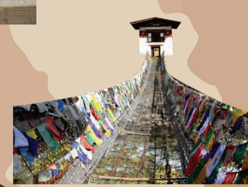
Cast iron bridge
